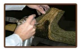
11. Using a fine nozzle spray gun, spray the char areas with the UCL Spray Stain.
